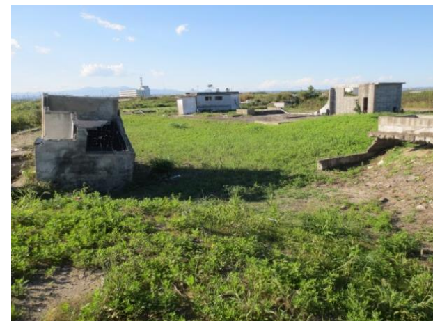
Ruins of the Great East Japan Earthquake: Residential Foundation
