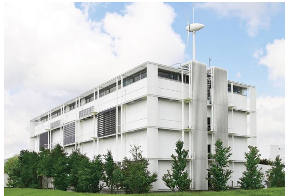
Photo.5 Fire-Resistance Test Facility
