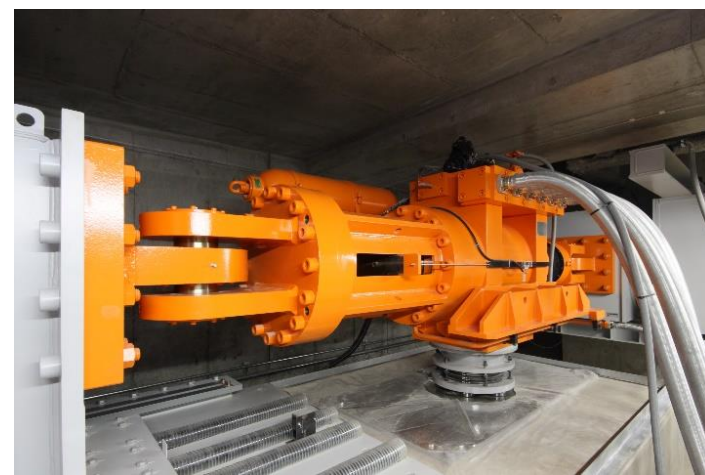
Photo.2 Super Active Base Isolation System Installed in Techno-Station Obayashi Corporation
