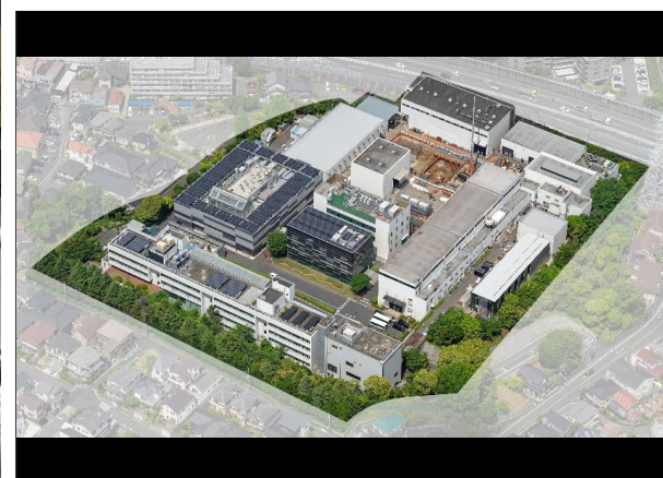
Photo.3 Taisei Advanced Center of Technology (TAC.T) Taisei Corporation
