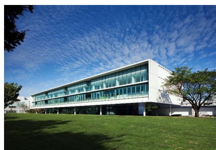
Photo.1 Main Building (Techno-Station) Obayashi Corporation
